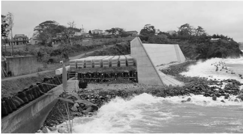
Figure 3 An Example of the Sea Wall Construction in Kesennuma City
